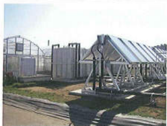
●太陽熱の吸熱板と放熱板、温水や冷水を溜める蓄熱槽●
